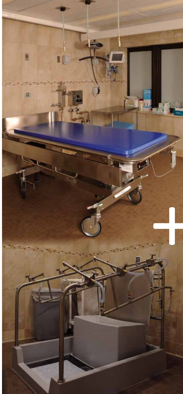
[ABOVE] The main tub room features “lay down” showering to provide head-to-toe care. A hydraulic trolley, ceiling and extremity lift help safely move and position patients. There is also a special tub room for infants and toddlers. All Burn Center rooms have monitoring capabilities. [BELOW] The sit-down shower area is for burn patients who are able to sit up for their wound care. It’s also a transitional area for patients to bathe and begin participating in cares before they are ready to shower on their own in their private rooms.
